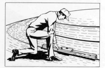
Use carpenter's level mounted on a 2 by 4 to lay out contour line.
